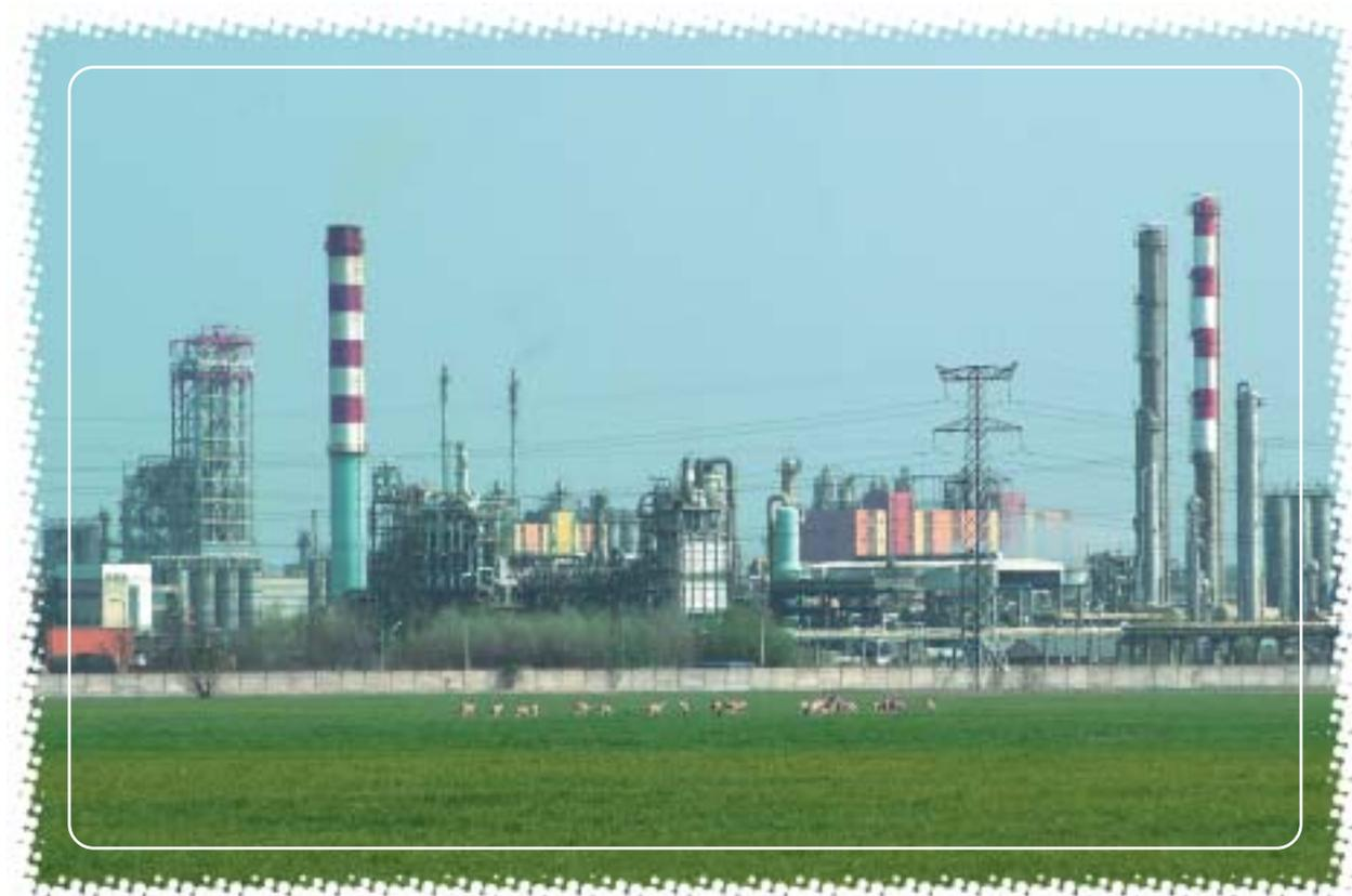
Flue gases exiting the stacks of the pyrolysis furnaces at the olefin plant account for most of the emissions.
